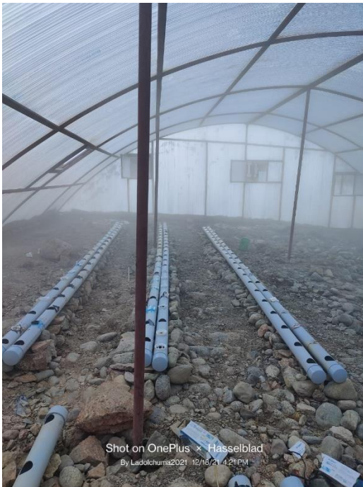
Figure 6: rusting due to the steam inside.
