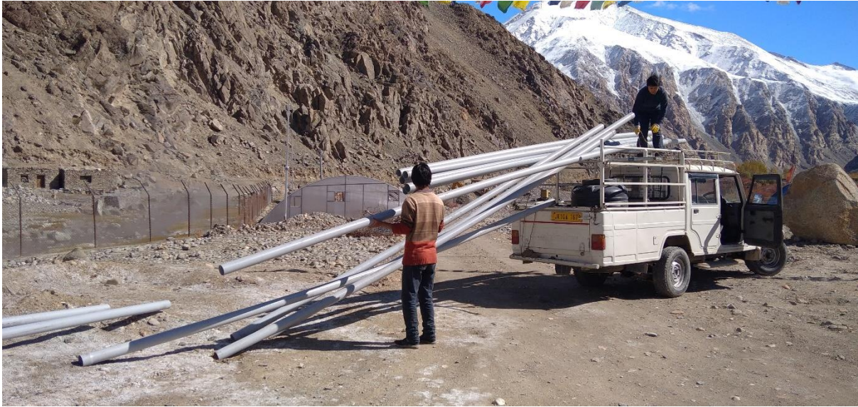
Figure 4: pipes for the soilless cultivation.
