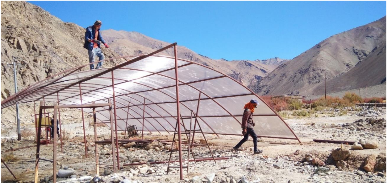
Figure 3: start of construction of the greenhouse.
