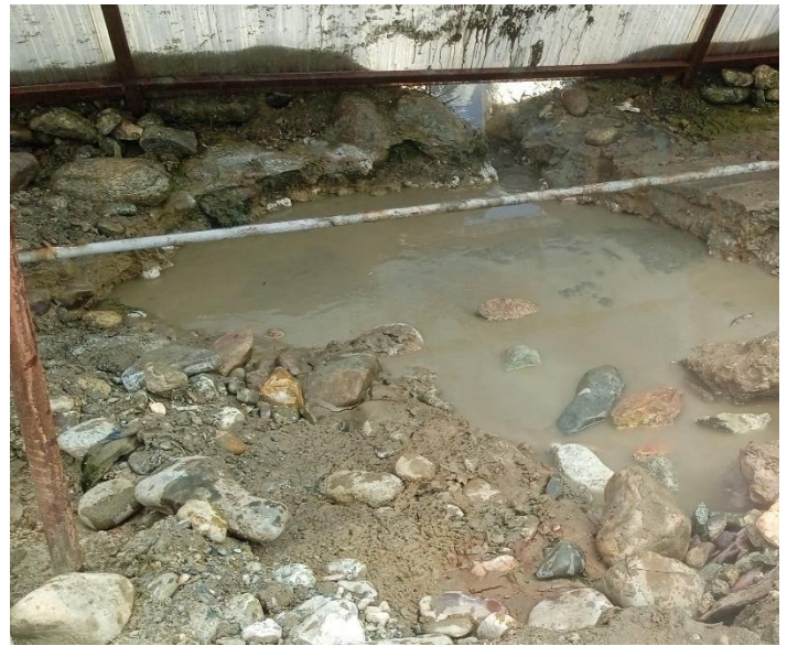
Figure 5: hot water pool inside the greenhouse which resulted in rusting.
